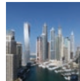
DUBAI Saving energy in air conditioning systems
